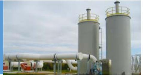
Perry Fiberglass Biotrickling filters are vertical or horizontal —oriented vapor-phase bioreactors filled with an inorganic media featuring 100% recirculation. The filters' unique design can address high concentration of H<sub>2</sub>S odors in areas where space is at a premium— offering a shorter retention time and treatment of higher air volumes than conventional biofilters. They can also treat high concentrations of VOCs and ammonia, and be chemically augmented when needed.
