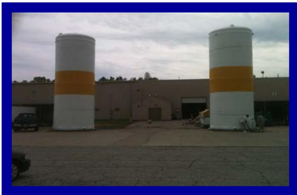
Shown above: Made to order Sodium Hypochlorite and Sodium Hydroxide Chemical Storage Tanks.
