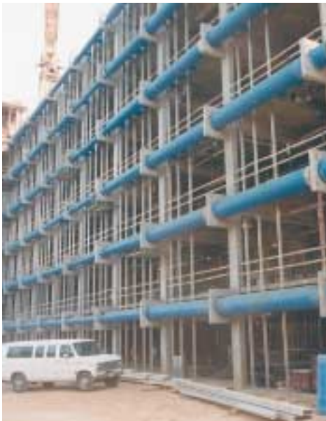
Left: Duct installation during construction Top Right: Close-up of round supply duct Bottom Right: Finished project
